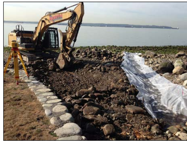
Image 2. Temporary redirection of creek flow and initial channel excavation.
