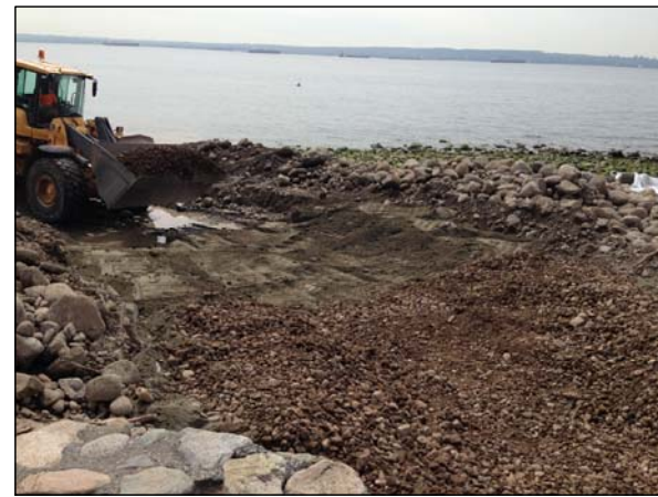
Image 3. Placement of clay/till sealing layer and 15cm minus filter rock.
