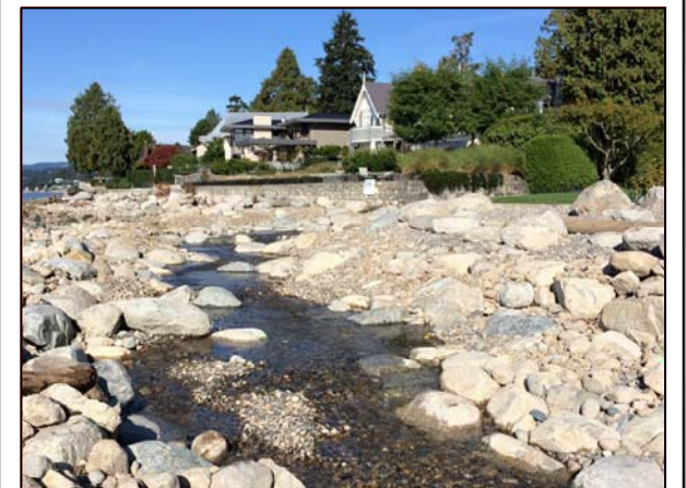
Image 7. After Rodgers Creek estuary enhancement. Note addition of large boulders and stream complexing when compared to Image 5 above.
