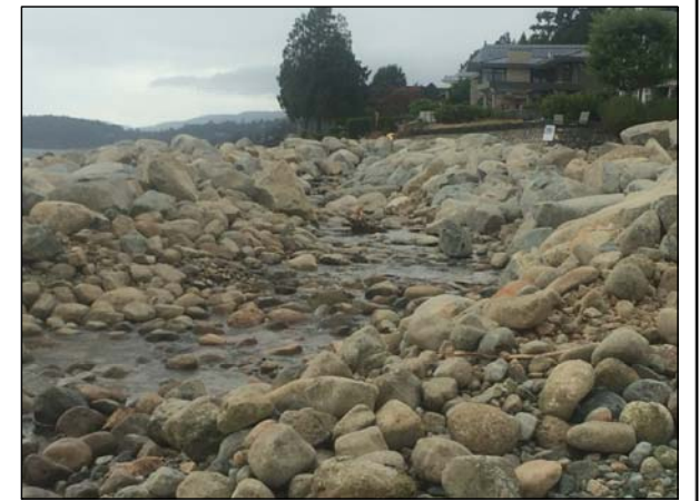
Image 5. Completed base of channel ready for creek complexing.
